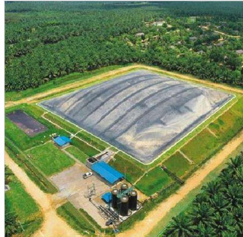
Biogas / renewable energy
